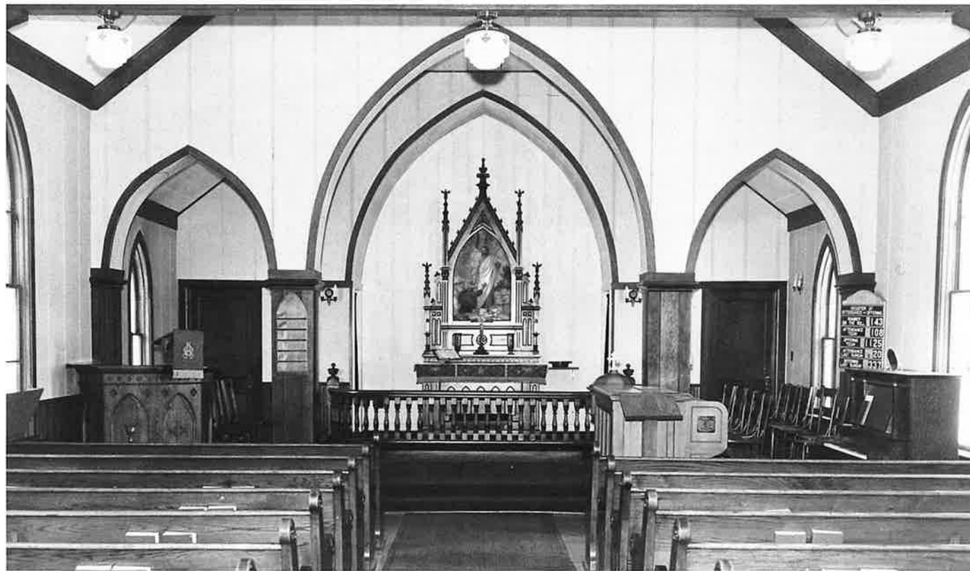
An interior view of the first church in 1962.
